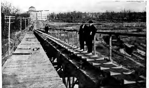
FIG. 2.—INTERIOR TROUGHING AND CARRYING BELT.
